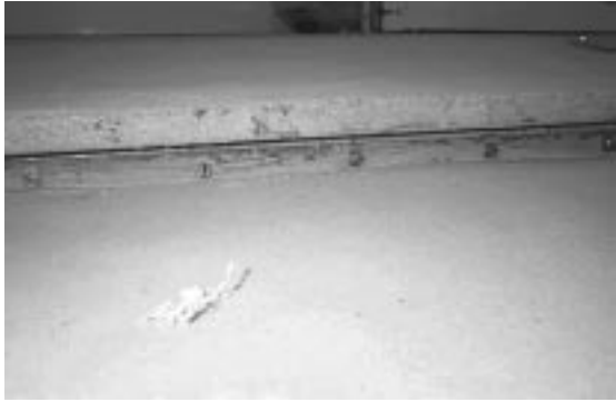
Figure 1. Water nozzles used to wash the manure from the gutter portion of the pen.
